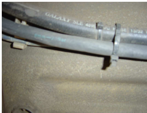
Figure 3 – Diesel & vegetable oil lines
